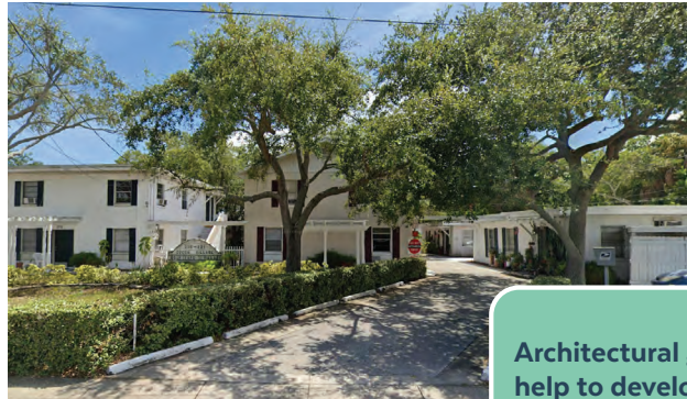
Cocoa Village Existing Garden Apartments
