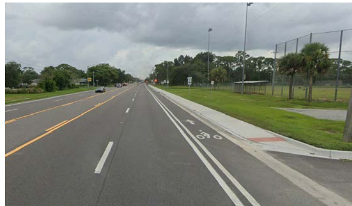
FDOT is planning pedestrian crossing improvements for Fiske Blvd to safely connect pedestrians to public open spaces
