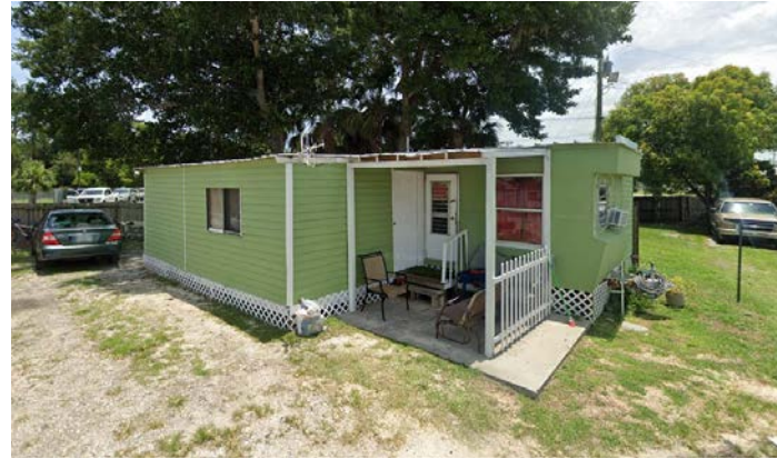
Some mobile homes lack accessible connections
