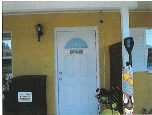
Not shuttered or labeled as impact rated
