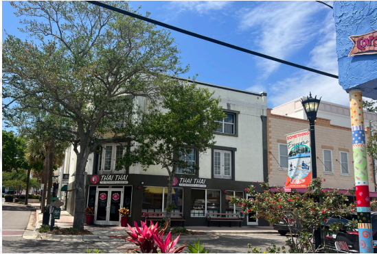
Thai Thai NW Corner of Delaney Ave and Harrison St.
