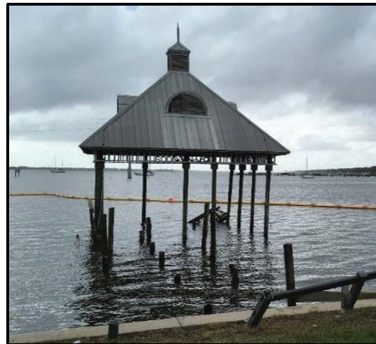
2017 Hurricane Irma Damage
