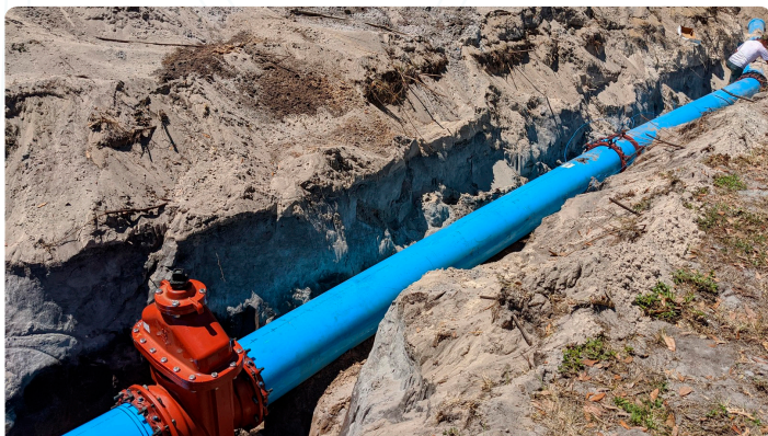
City of Davenport Water Main Replacement
