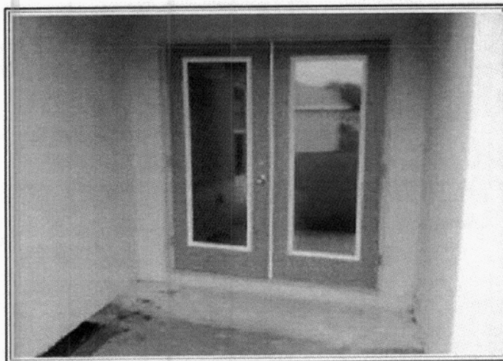
Covered Porch / Open Patio
